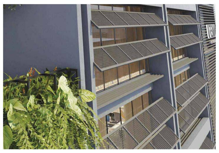
The double skin facade and substantial presence of vegetation further reduces heat loads.
