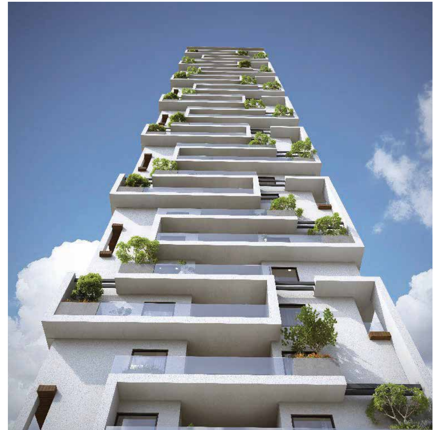
Extruding residential units at Myscape – Isle of Sky Cubical shaped balconies are staggered vertically on elevation to ensure natural lighting and plantation on every floor.
